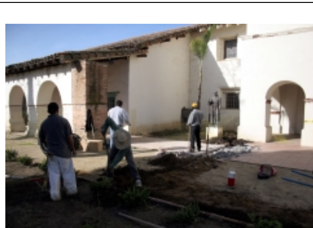
Trenching operations exposed the foundations to the Victorian bell tower and revealed that the Serra statue was installed immediately atop said foundations. Photo © Ruben G. Mendoza, 2006.
