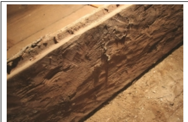
The redwood planks that compose the Convento floor were harvested from the Santa Cruz Mountains, and generally measure some 22 linear feet. Note ship lapped and adzed underside of plank. Photo © Ruben G. Mendoza, 2006.
