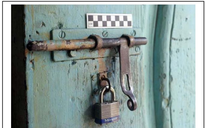
Image of slide-bolt from the Mission Hardware Survey collection. Photo © Ruben G. Mendoza, 2007.
